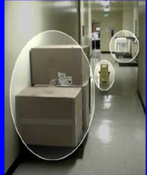
Obstructed exit route
