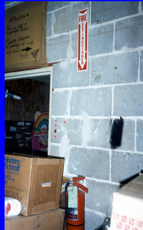
Blocked extinguisher
